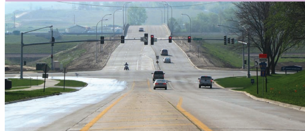
Economic growth is expected to get a boost in the Floyd Blvd/Outer Drive area and the north side with the new Outer Drive Bridge opening.
