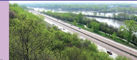
Improvements continue this summer on I-29.
